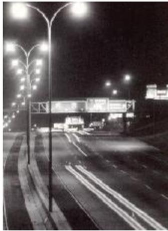
**A freeway section with continuous lighting has overhead lighting at the interchanges and between the interchanges.**
