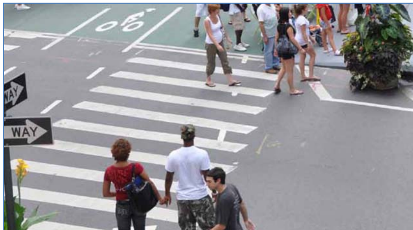
FIGURE 3 High Visibility Crosswalk in New York City
